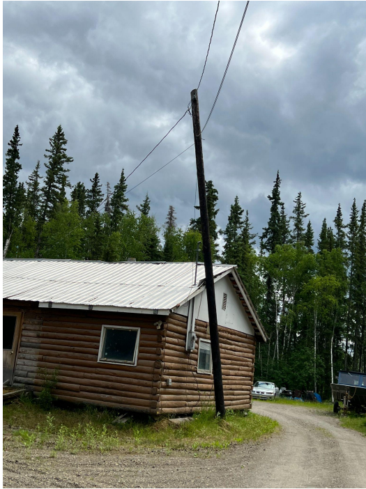
Tilting power pole in Galena (Logan Borger, 2022)
